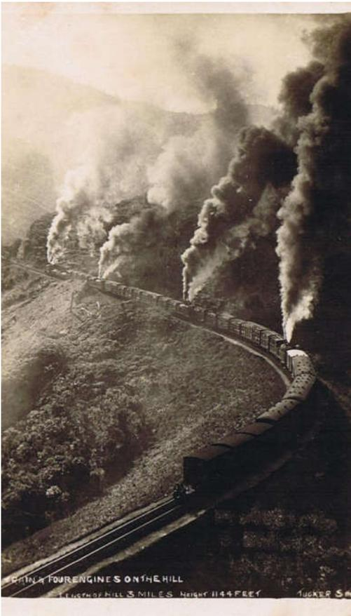
It still took 4 Engines to haul the train over the hill and when they headed down the brakes were working overtime and had to be replaced each trip.
